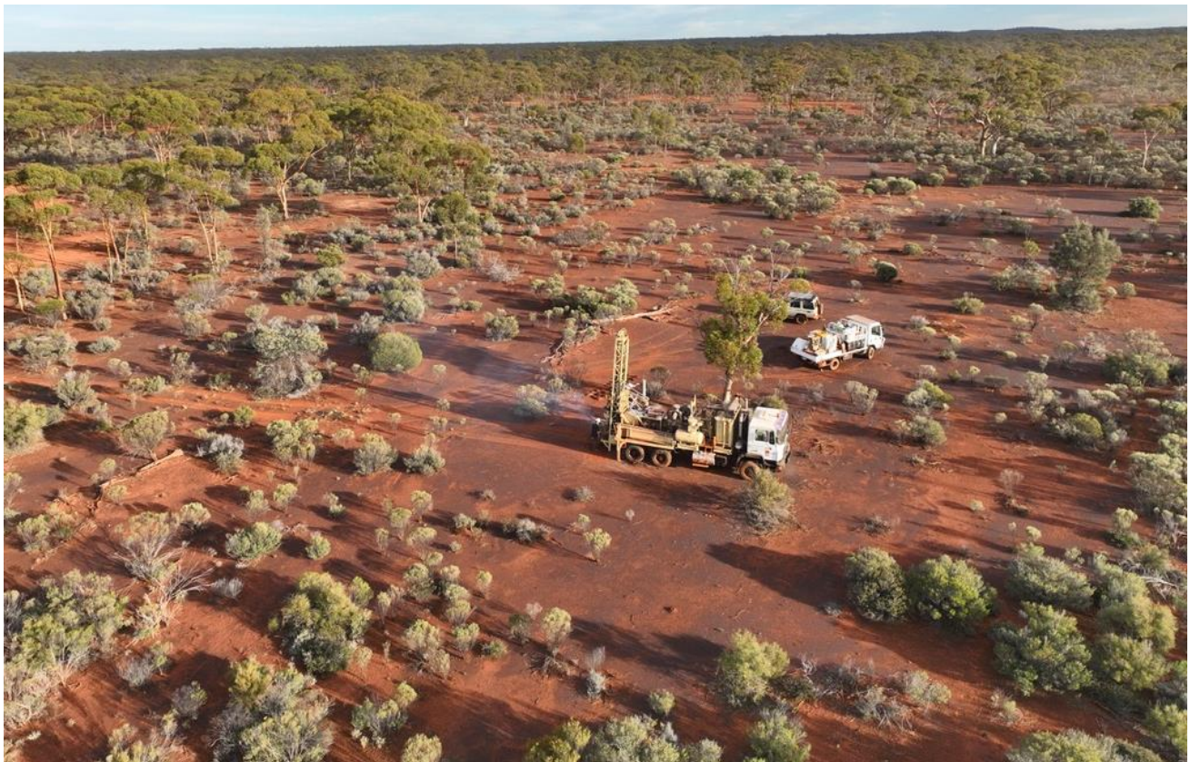
Figure 2: Australian Aircore Drilling AC rig on site at the Northern Zone Project
